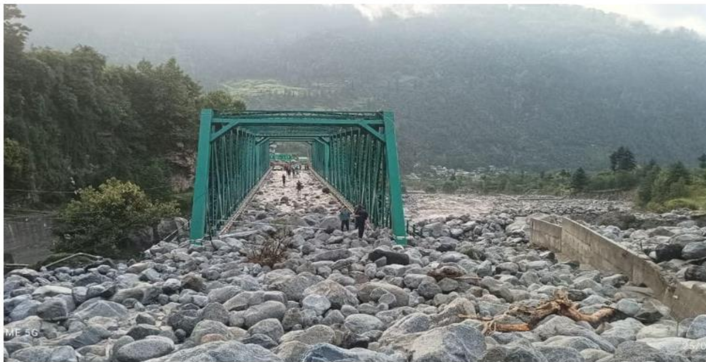
The Manali-Leh Highway blocked with rocks after heavy rainfall in Palchan. Photo provided by Rohit Prashar
